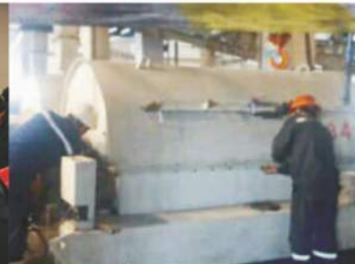
Installation of Centrifuge
