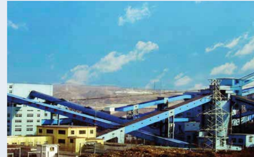
Shenhua Group Qilian Tower Coal Preparation Plant
