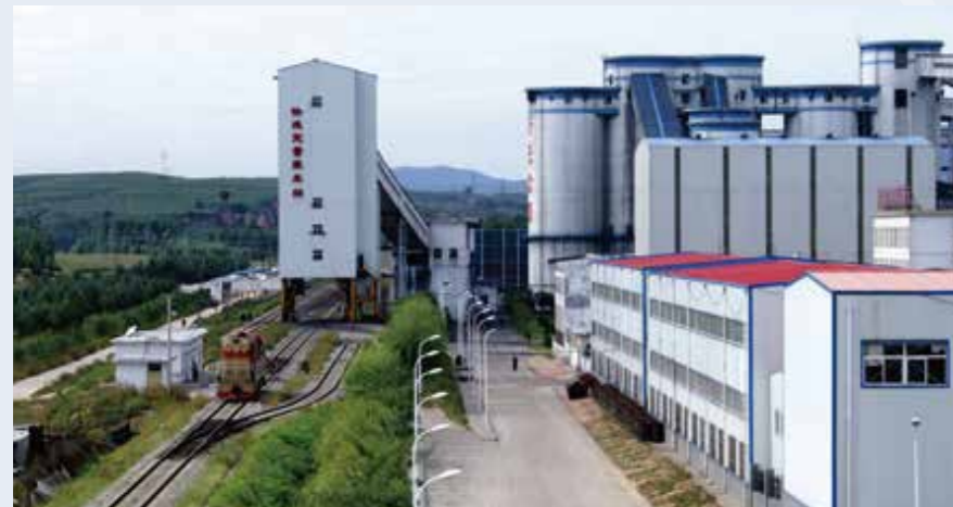
Singapore Dollar Coal Preparation Plant
