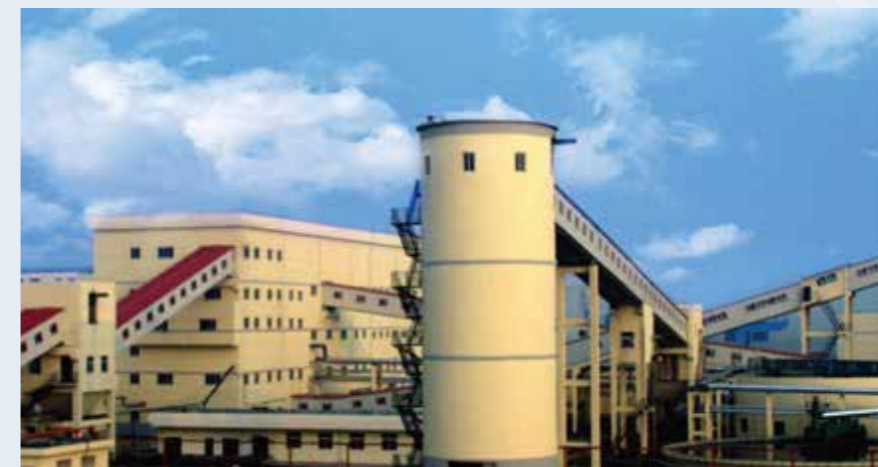
Northern Anhui Coal Power Money Camp Coal Preparation
