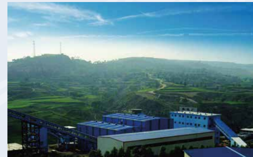
Fenxi Mining Group Shuguang Mine Coal Preparation Plant
