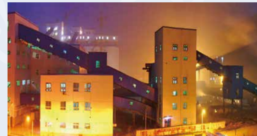
Huangling Coal Preparation Plant of Huangling Coal Industry Group
