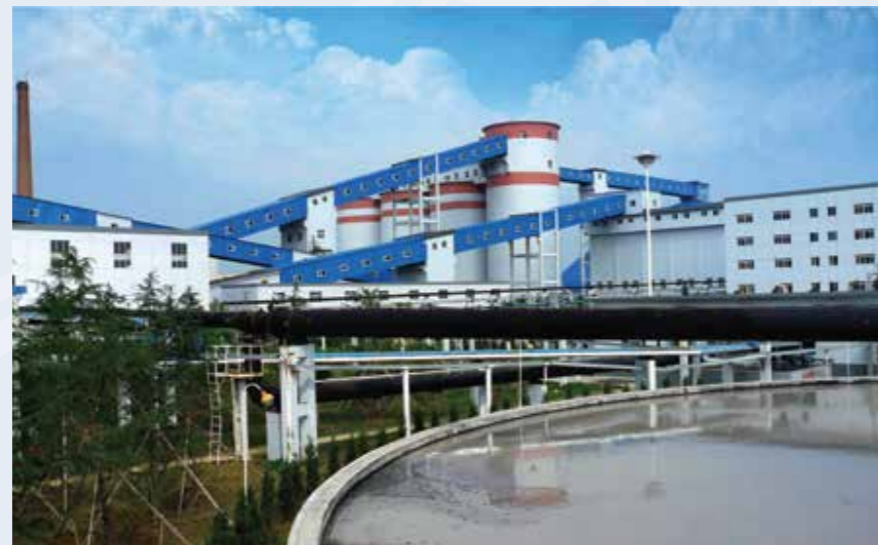
Huainan Mining Group Dingji Mine Coal Preparation Plant
