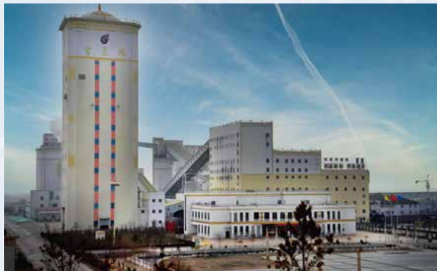
Yingpan Trench Coal Preparation Plant
