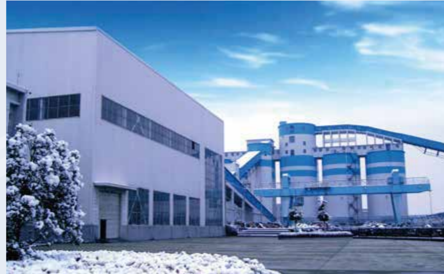
Huainan Mining Group Panbei Mine Coal Preparation Plant
