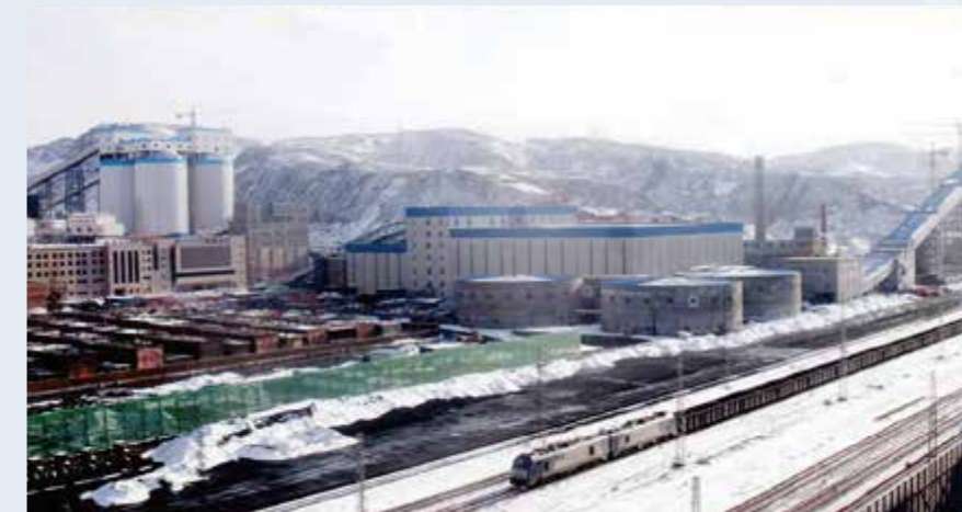
The largest slant hook coal preparation plant in the world by annual production at that time
