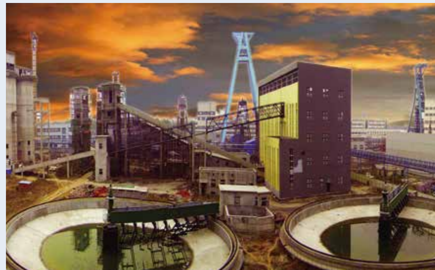
Huainan Mining Group Gubei Coal Preparation Plant
